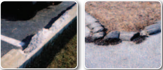
Concrete curb cannot survive even a short period if it is not backed up by soil. Berm always fails the snowplow test.
