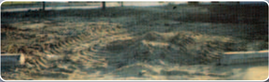
Here, a section of precast curb was completely pulverized by construction equipment at a shopping center.
