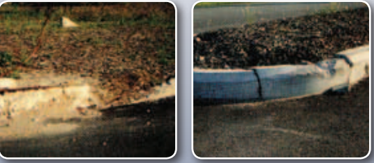
The effects of impact are obvious in these examples of precast curb installed less than three years ago.
